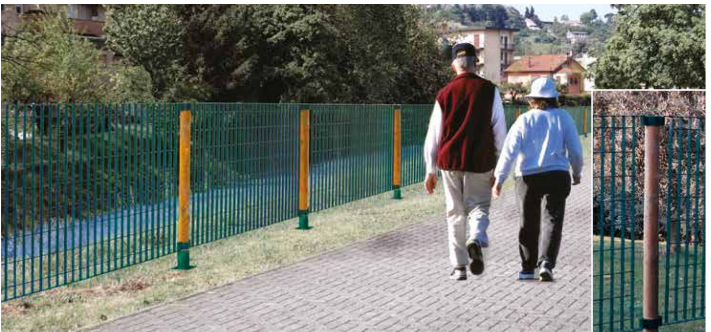
PROJECT: to secure embankment fencing near a pedestrian path
